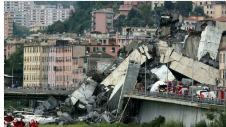
The collapsed Morandi Bridge in the Italian port city of Genoa, Italy, 14 August 2018. REUTERS/Stefano Rellandini
