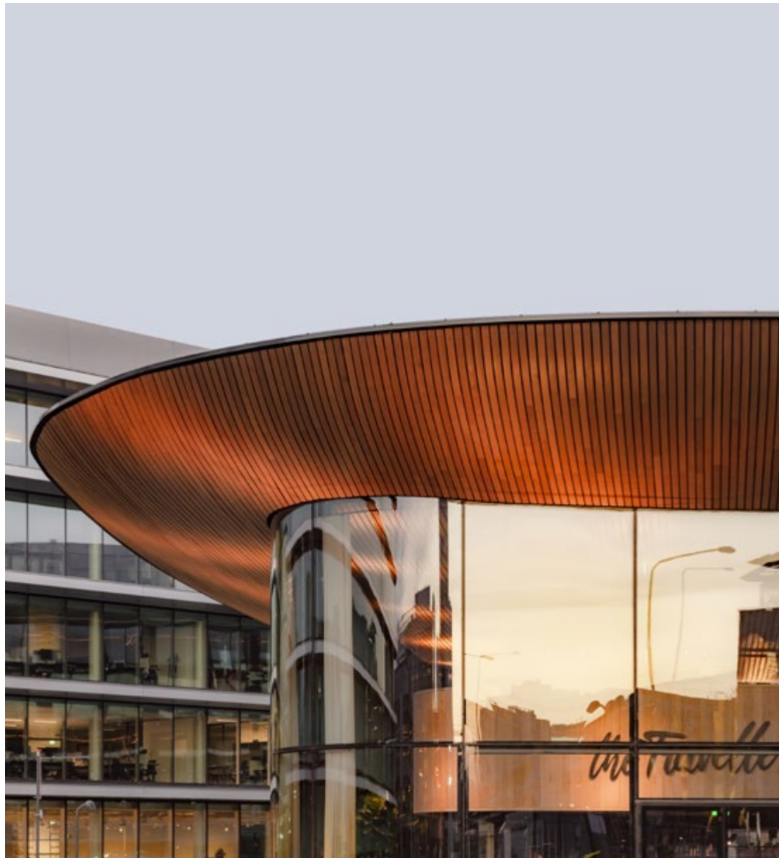
The larch roof with its double curvature
