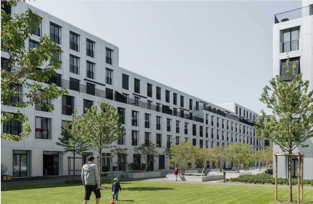
Source: Implenia AG
