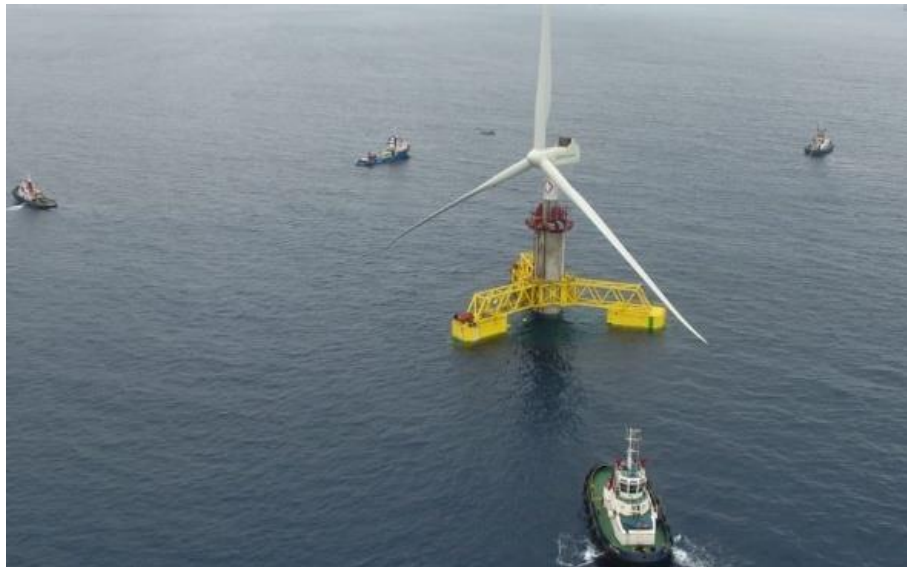
The ATOMS platform (top) uses the Coupling Ring System (CRS) already developed and proven as a tool for installation of ELISA GBS units (bottom).
