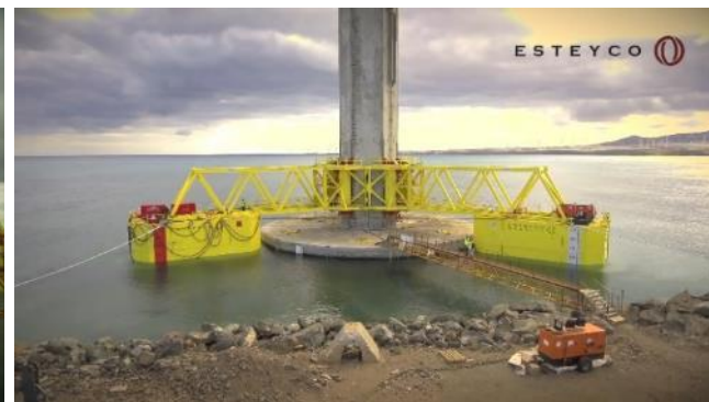
The ATOMS platform uses the Coupling Ring System already developed and proven as a tool for installation of ELISA GBS units as shown in the TIM in pictures above where it is depicted in the ELICAN project..
