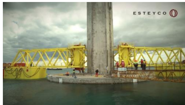
The ATOMS platform uses the Coupling Ring System already developed and proven as a tool for installation of ELISA GBS units as shown in the TIM in pictures above where it is depicted in the ELICAN project..
