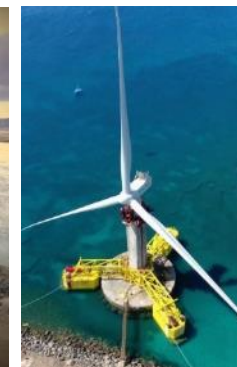
The ATOMS platform uses the Coupling Ring System already developed and proven as a tool for installation of ELISA GBS units as shown in the TIM in pictures above where it is depicted in the ELICAN project..
