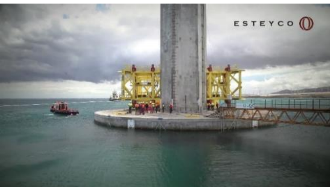
The ATOMS platform uses the Coupling Ring System already developed and proven as a tool for installation of ELISA GBS units as shown in the TIM in pictures above where it is depicted in the ELICAN project..
