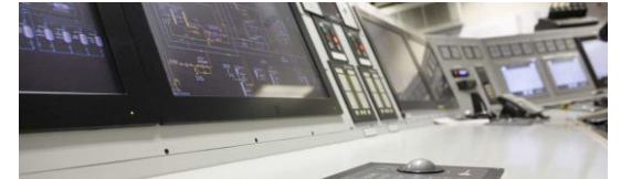
Screen in bridge
